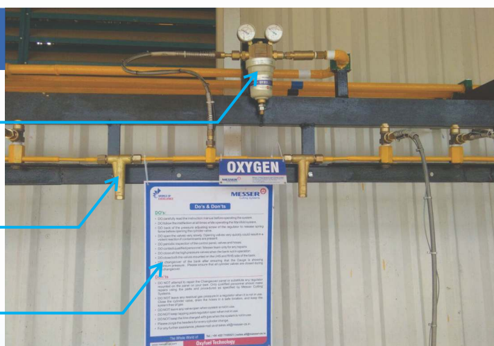
2x10 Oxygen Cylinder Manifold with U13 regulator & F11 filter
