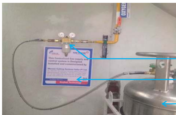
2x10 Oxygen Cylinder Manifold with U13 regulator & F11 filter
